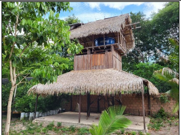
Photo 11: ACRAA's headquarters building (under development), also the water tower for the property. An artesian well is located below the tower providing essentially unlimited water. Photo Jan. 2024.
